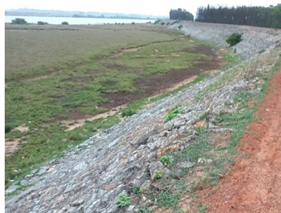
Fig. 4: Construction of non-erosive stone wall
