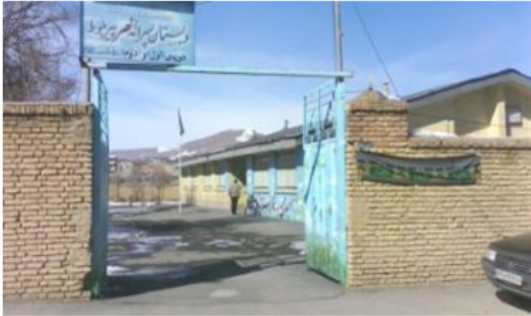
Fig. 6: the school exterior façade
