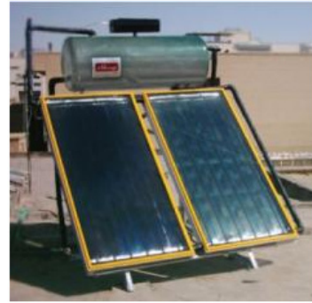
Fig. 7: the solar water-heater with a selective flat thermo-siphon model: T200
